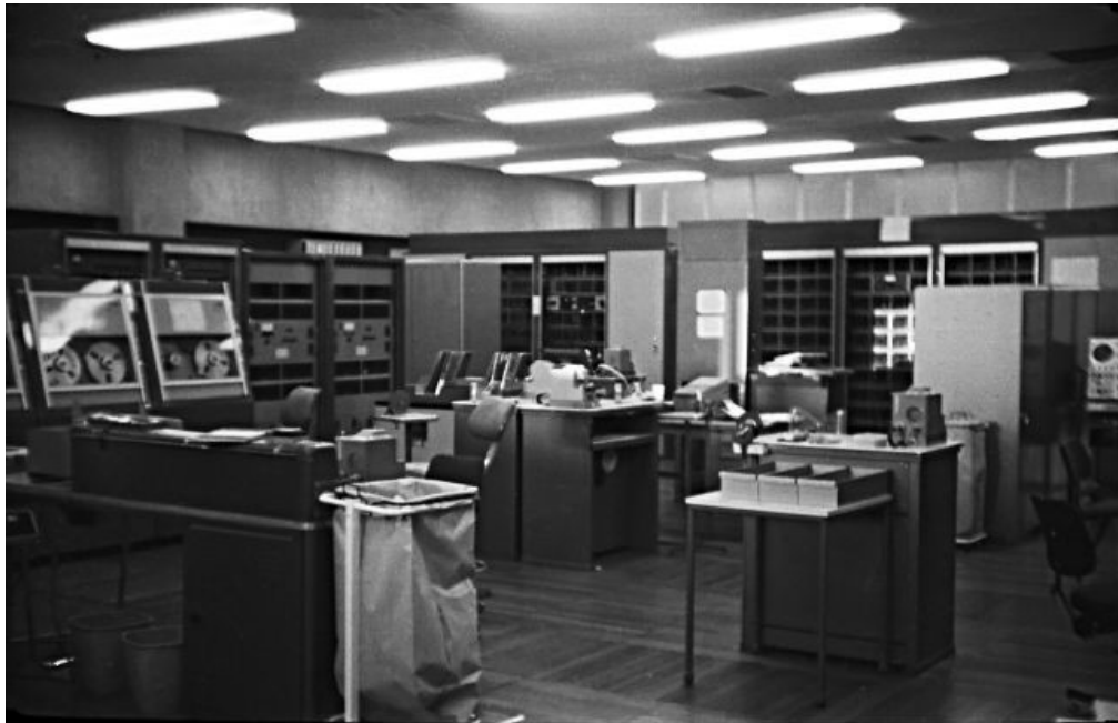
Figure A2. The final Titan configuration in its new machine room, some time after 1969.
