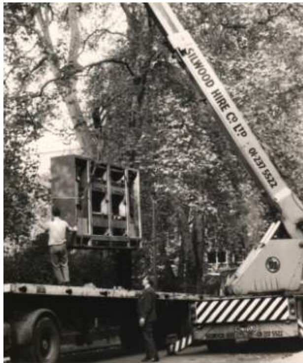
The computer was dismantled into cabinets weighting several tons each and varying in length from 8 to 12 feet.
