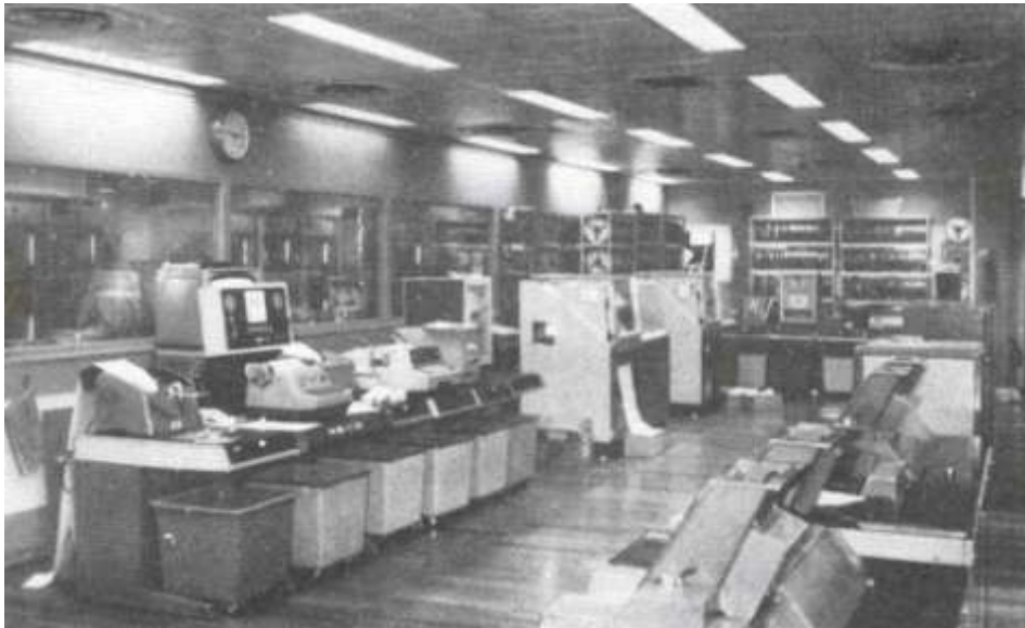
This photograph shows the main upstairs computer room where the actual work was done. The spiral stair case described by the author was in the adjoining left-hand small room
