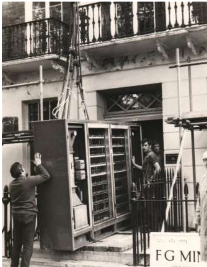
A view of one of the cabinets being taken through the front door. The building in which ATLAS was housed is scheduled as a building of historical interest and great care had to be taken not to damage the balcony or the fabric of the building
