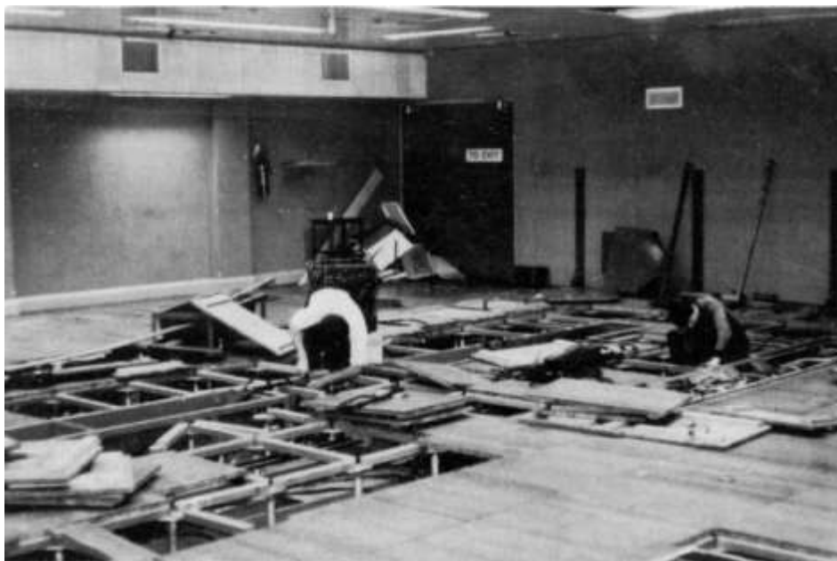
The downstairs room with its false floor, the computer finally removed and the engineers dismantling the cabling of which there was a considerable quantity. Large pieces of cabling had to be of a precise length so as not to upset the timing of the computer's operation.
